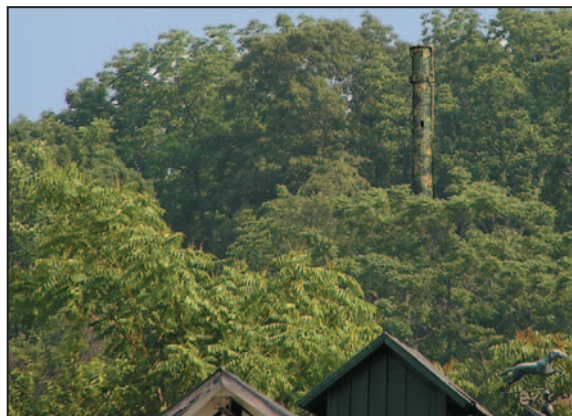
Invisible Towers' projects employ a number of camouflage solutions designed to engage community support for antenna sites.
